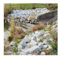
In late December of last year, we replaced the rocks (Rip Rap) around the inlets to the pond. This was needed due to erosion around the inlet pipes. Continued erosion would result in silt accumulating in the pond and is also unsafe due to a trip hazard. The cost of this project was \$5800 which was covered from reserve funds.
